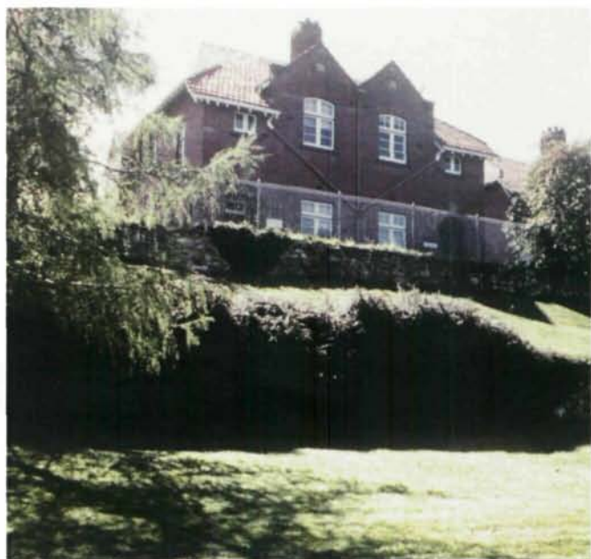
Built in 1913 as sergeants' married quarters, now 'Despard House' and 'Chesney House'.
