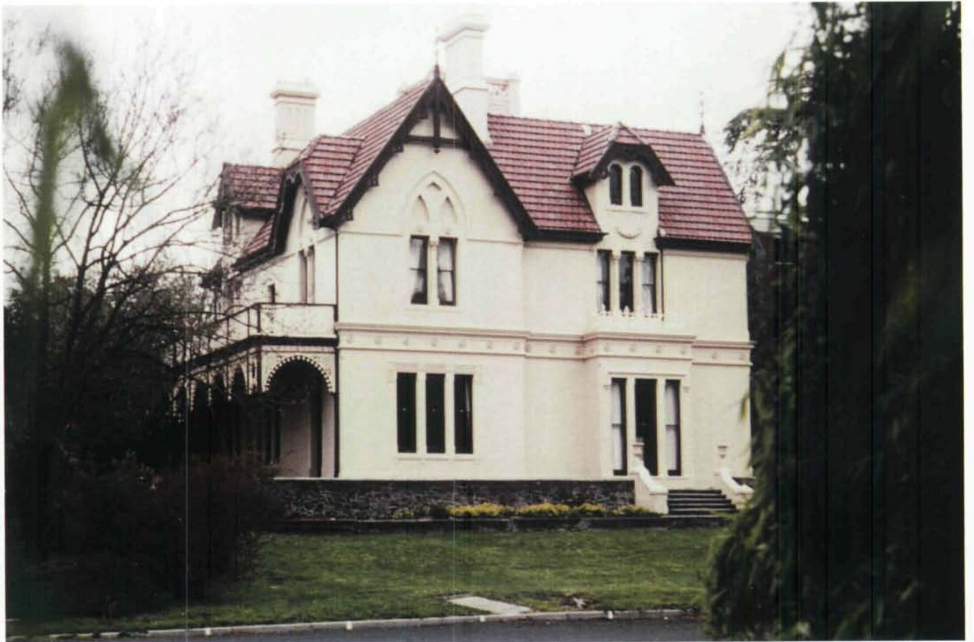
Beaumaris House. At one stage of its history, the front grounds of this property housed Hobart's first zoo.
