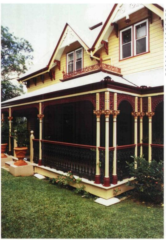
The verandah was originally a very generous space large enough to entertain on a fine scale. The construction consisted of a timber framed roof and floor structure with cast iron columns, balustrades and decorative details. The ceilings have been lined with wide beaded timber boards. The verandah was finished in an appropriate colour scheme and by hanging two striped canvas blinds, as seen in historic photographs, is protected from the sun.
