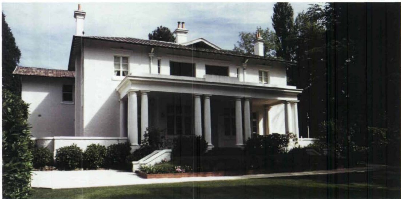
This photograph of Bridges House was taken just prior to the recent sandblasting of the exterior. This process allowed the external walls to be restored to the original ochre wash colour, rather than the white of the last few decades, and to restore the original colour configuration.
