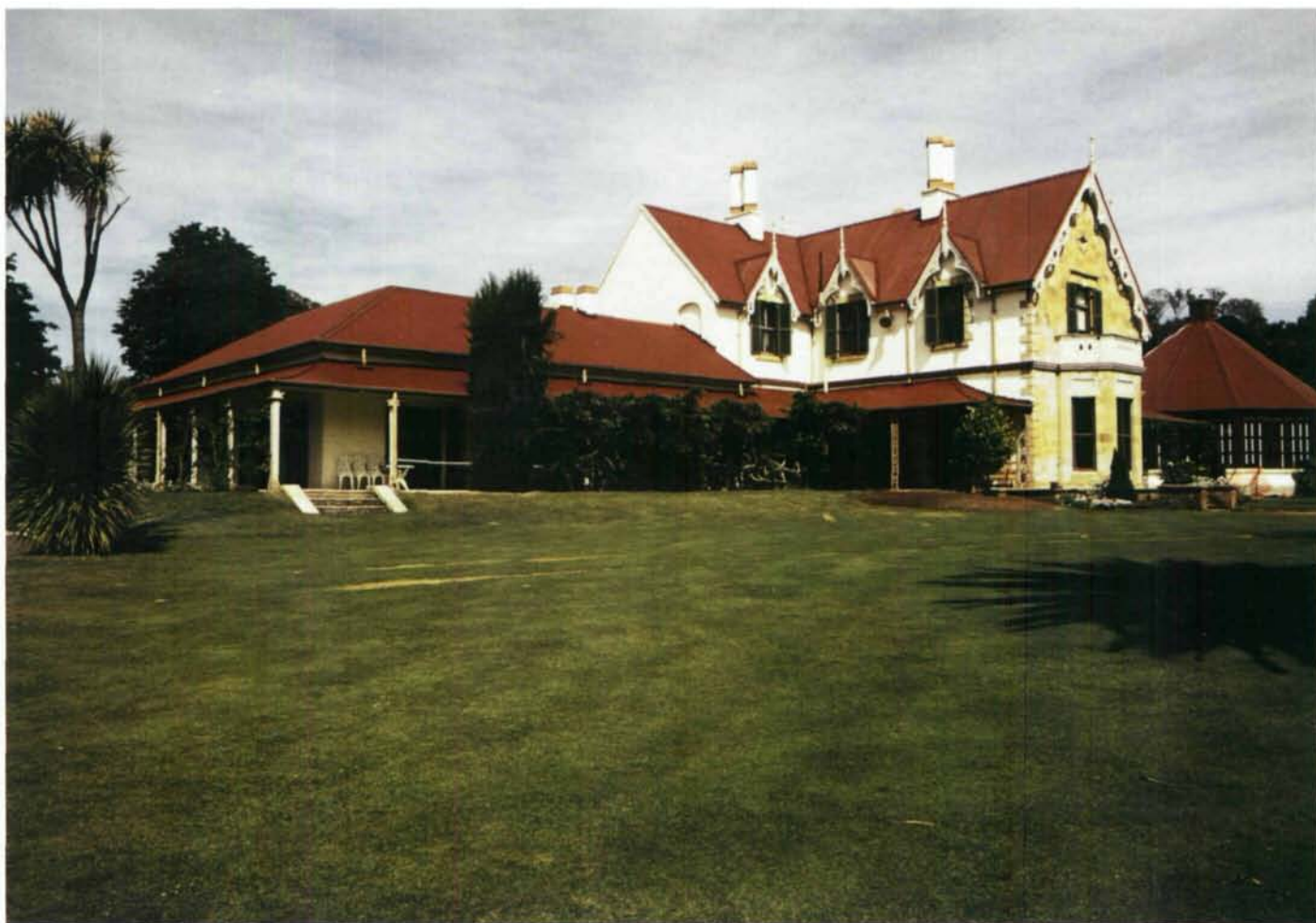
Duntroon House is the oldest building in Canberra and, along with its gardens, is listed by the National Trust and on the Register of the National Estate. Its architectural history is displayed in the main hallway.
