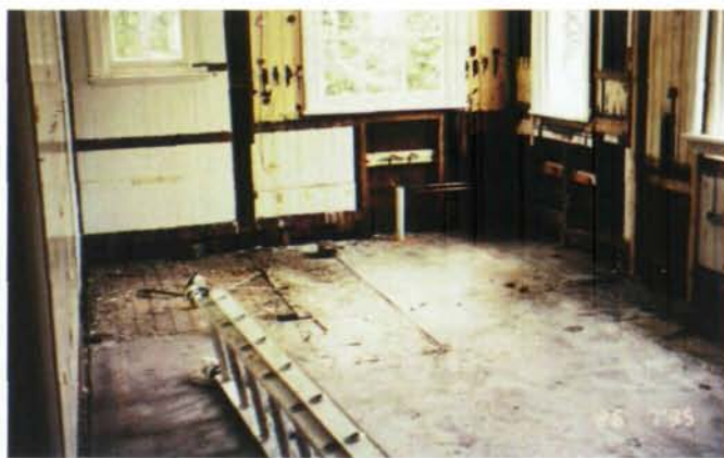
Extensive renovation work being undertaken at 7 Morgan Street, HMAS Creswell.
