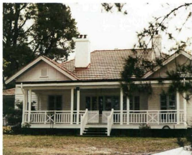
An overall effect of the College is of well mannered architecture, carefully detailed with Georgian-derived joinery, slatted timberwork railings and brackets, and expressed rafters at the eaves. The residences maintain this excellent timber vocabulary, though their verandahs and asymmetrical bungalow form link them with typical timber residences of the Federation period.
