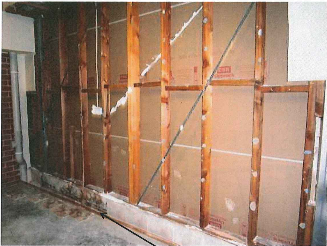
Location of entry point at slab joint in garage
