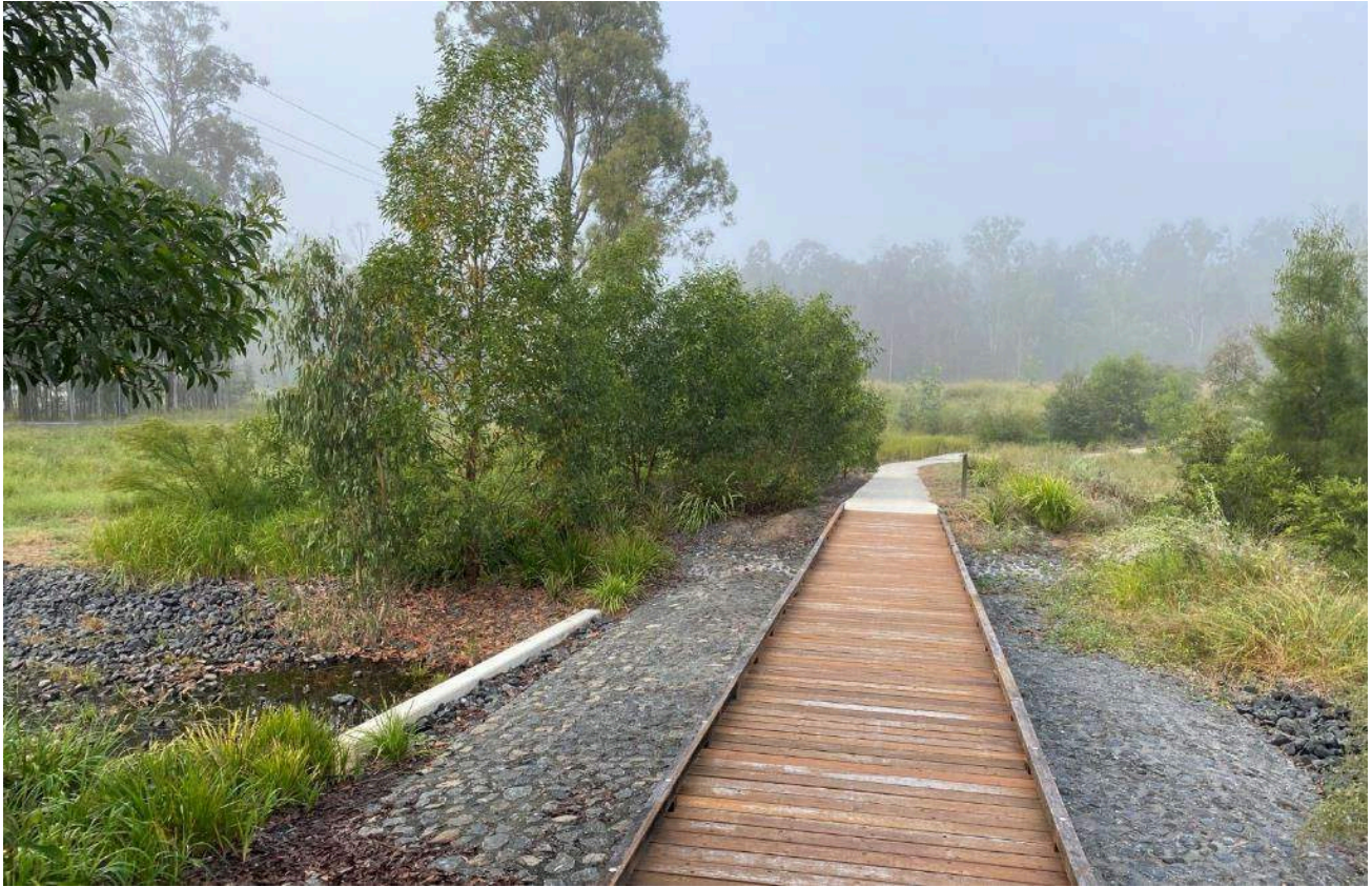
Photo 3: Pedestrian bridge over culverts within Stage 1 rehabilitation area – May 2021
