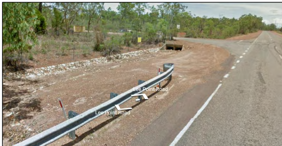
Figure 4-1 Former RAAF Facility Entry Road (Ref: Nearmap 2016)
