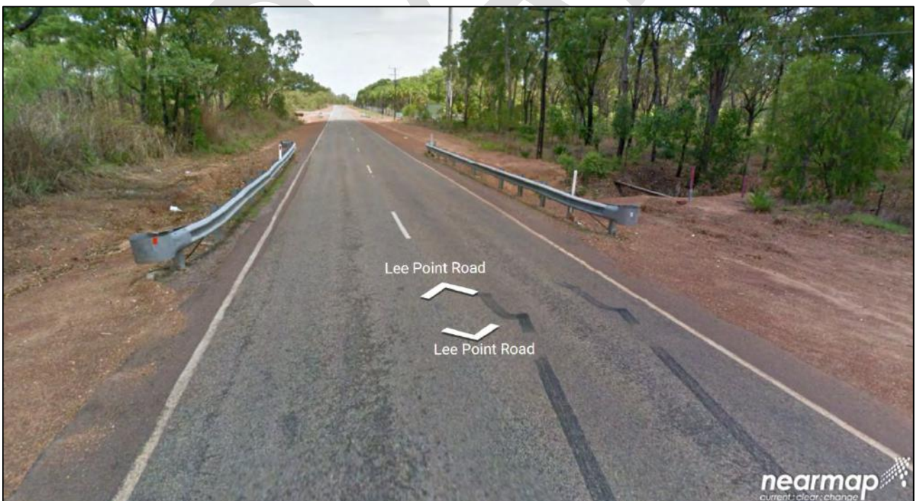
Figure 11. Culvert cross of Lee Point Road 115m south of the Lee Point Resort (Nearmap 2016).
