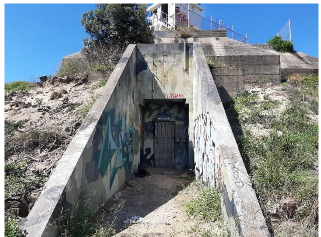
Figure 30 – Tunnel entry, Item A0037.
