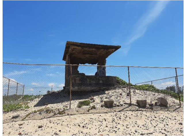
Figure 10 – View of northern searchlight in poor condition, with fencing to attempt to prevent further damage.
