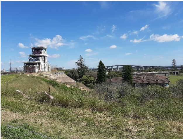
Figure 13 – Observation Tower, Item A0036, junior sailors accommodation and Stockton bridge in background.
