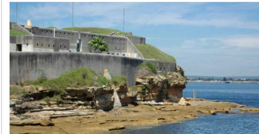
Below: view of concrete wall and structures, Bare Island Fort. Source: La Perouse Museum
