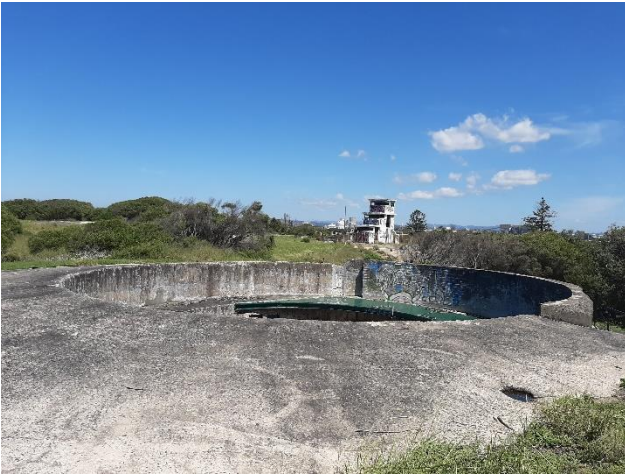
Figure 19 – View from No.2 Gun Emplacement, 9.2 inch guns, Item 27, towards Observation Tower.
