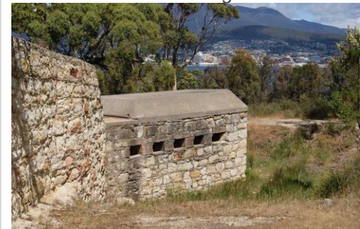
Below: Kangaroo Bluff, tunnel entry structure. Source: Australian Heritage Database.
