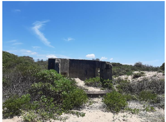
Figure 24 –.Southern searchlight 9.2 inch guns, in dilapidated condition, Item 103.
