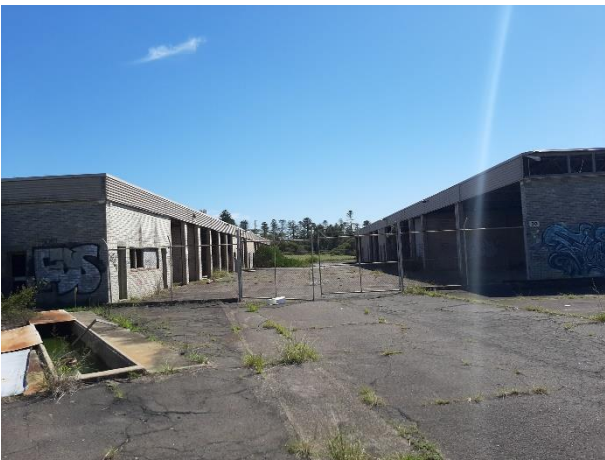
Figure 32 – View north towards the Transport Naval Stores (Item A0030), with Item A0019 to left of frame.
