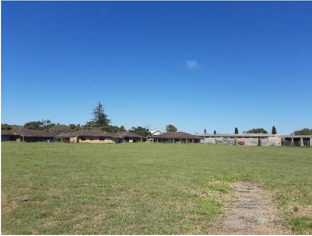
Figure 9 – View west towards naval store sheds and junior accommodation buildings.
