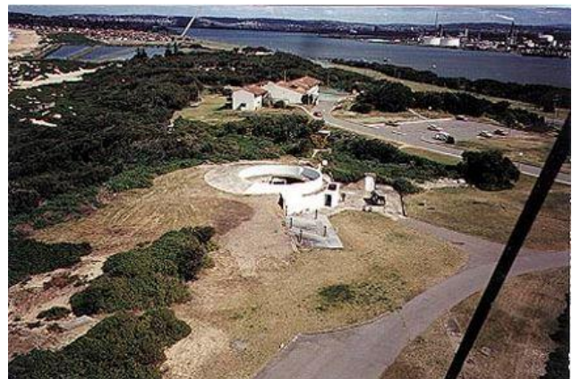
Figure 59 – Aerial view, undated. Multistorey barracks to left, background, since demolished.
