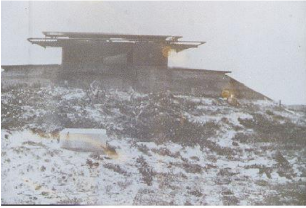
Figure 44 – battery observation post, 1929, Fort Wallace
