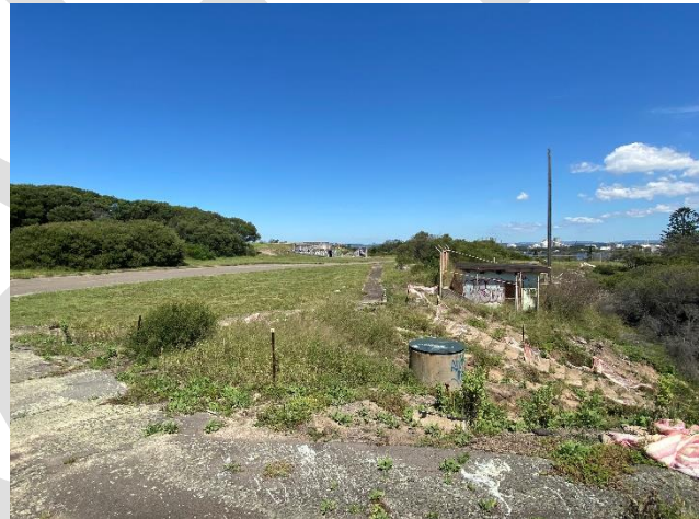
Figure 67 – Internal view corridor to gun emplacement to south.
