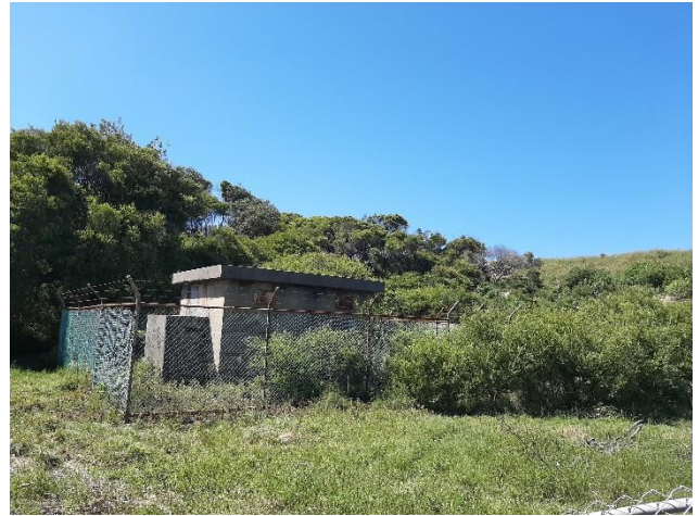
Figure 28 – Engine Room, Northern Searchlight – 9/2 Inch guns.
