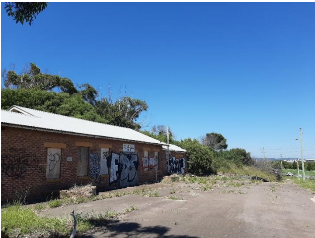
Figure 23 – Admin Building, Engine House 6 Inch Guns, Item A0007.
