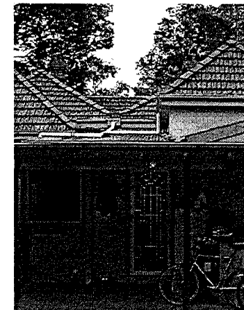
Valley gutter detail
