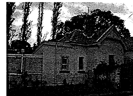
NE corner view
