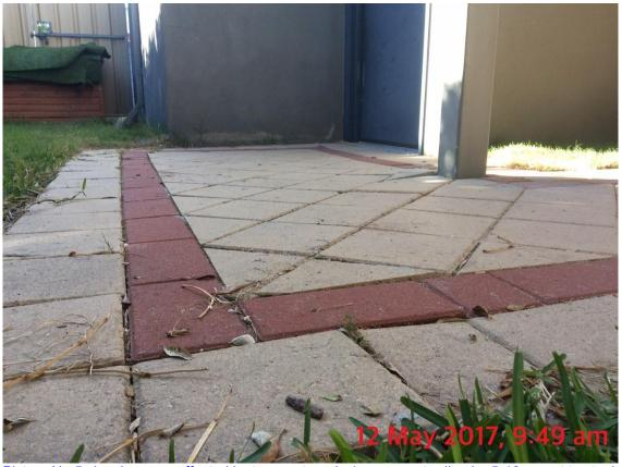
Picture No.5 showing area affected by tree root, and x1 paver protruding by 5-10m next to steel post
