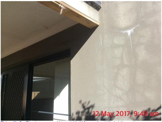
Picture No.6 – Showing map cracking, paint bubbling, and sprinkler/misting system
