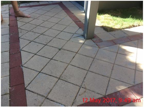
Picture No.4 – Showing area of paving affected by tree root
