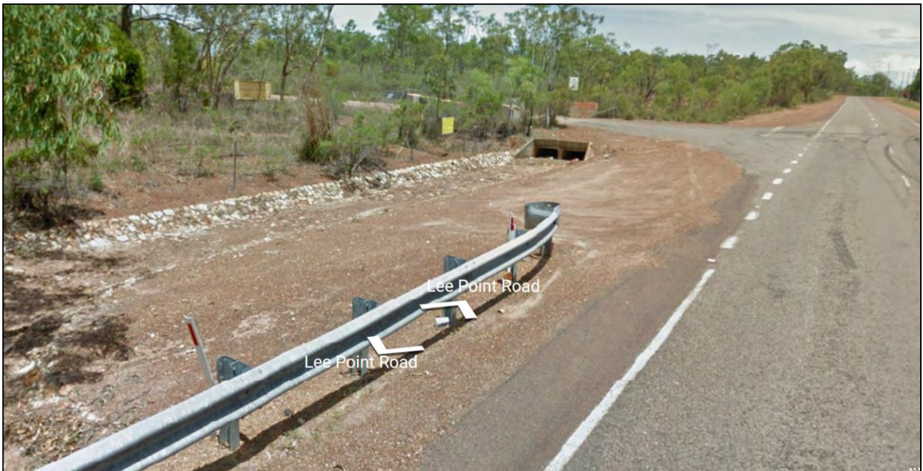
Figure 10. Entry road to 2CRU
