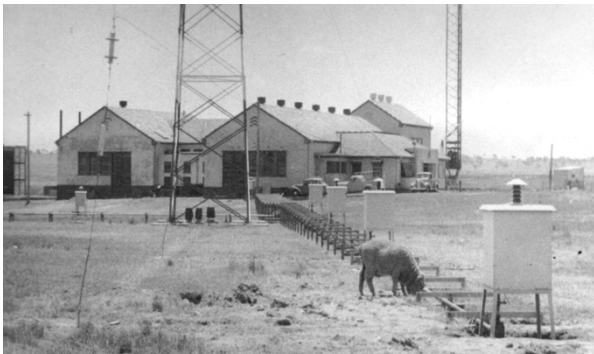
Figure 3.11 The transmitter building with sheep grazing nearby, pre-1941. (Source: Tremlett Collection from 2001 HA)
