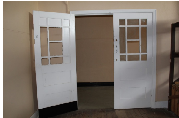
Figure 4.30 Smashed glazed panels in doors to room 32 (2018).
