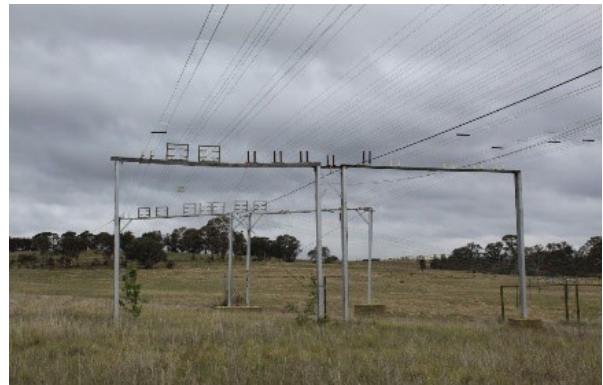
Figure 4.36 One of the remaining aerials on the site which connects to the first-floor aerial switching room, 2018.
