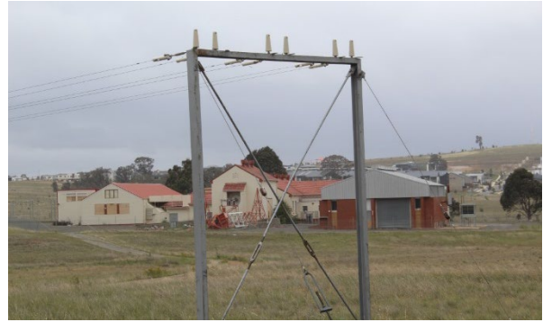
Figure 4.34 An example of the remaining aerials on the site, 20.
