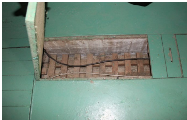
Figure 4.26 The subfloor service ducts (2018).
