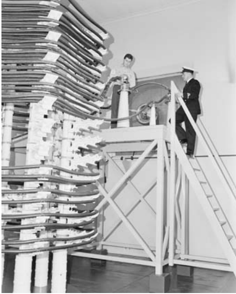
Figure 3.21 Aerial loading coil located in the helix room at the transmitting station, 1961. (Source: National Archives of Australia, A1200, 11139796)
