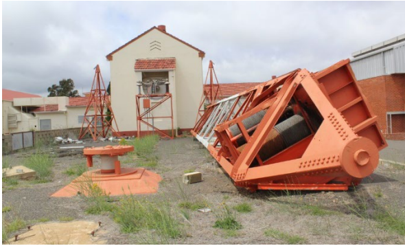
Figure 4.33 A portion of the 183m landmark towers that supported the aerial, dismantled and lying near the Helix Room, 2018.
