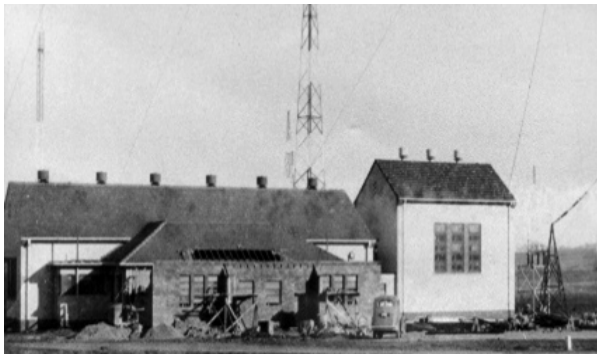
Figure 3.12 Construction of the 1941 extension at the front of the original entry and transmitter hall. (Source: Tremlett Collection from 2001 HA)
