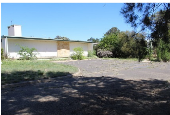
Figure 4.47 The Senior Sailors' Mess and accommodation building looking southeast, 2018.
