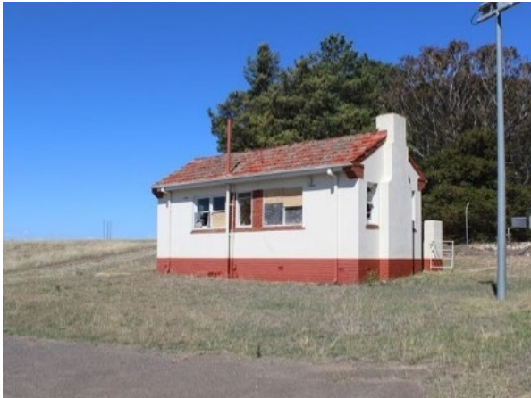
Figure 4.43 The guardhouse looking east. Note the partially ply infill windows, 2018.
