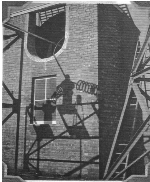
Figure 3.24 Bomb-blast proofing situated around the aerial feeder, at the northern wall of the Helix Room, before render 1942. (Source: Tremlett Collection from 2001 HA)
