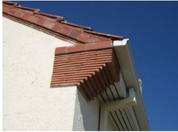
Figure 4.44 Decorative terracotta corbels on the guardhouse which are also featured on the earliest section of the transmitting building, 2018.
