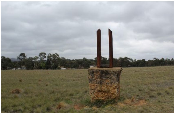
Figure 4.35 Example of the remains of original rhombic aerial base which would have supported timber poles, 2018.
