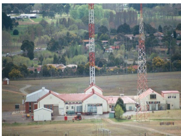
Figure 3.7 Transmitting station complex and adjacent aerials in 2000. (Source: 2001 HA)
