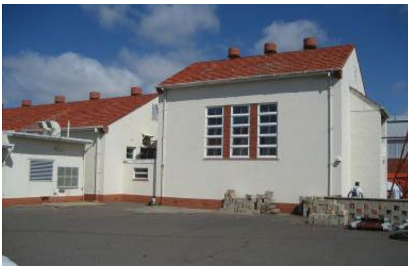
Figure 4.25 2008 photo showing the exterior of the helix room and the contrasting horizontal and vertical features of the window details. The window has now been boarded up for security measures.
