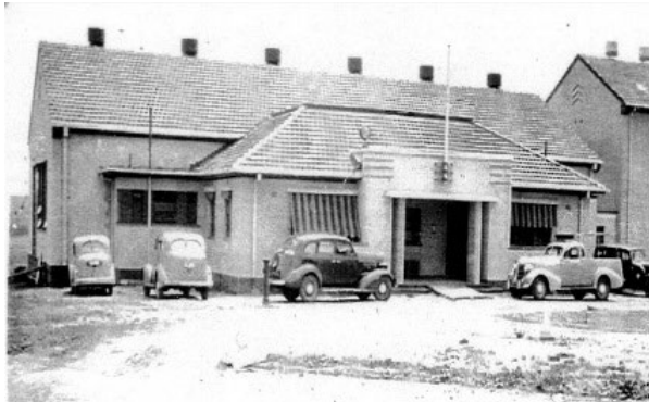
Figure 3.10 Main entrance to the transmitting building, c1940/1941. The helix room has been added to north. (Source: Historical Collection from 2001 HA)
