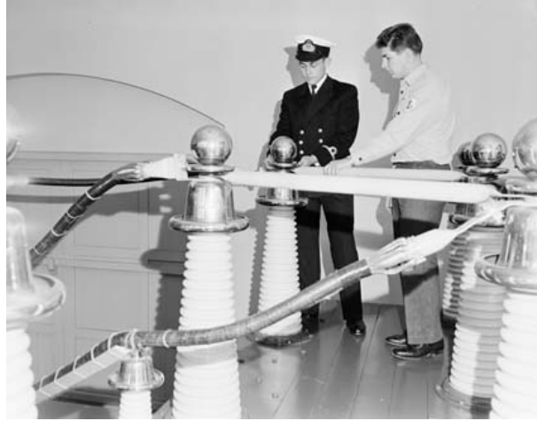
Figure 3.22 Connecting links of the loading coil between a transmitter and its aerial. The stainless-steel globes prevent corona discharge. (Source: National Archives of Australia, A1200, 11139799)
