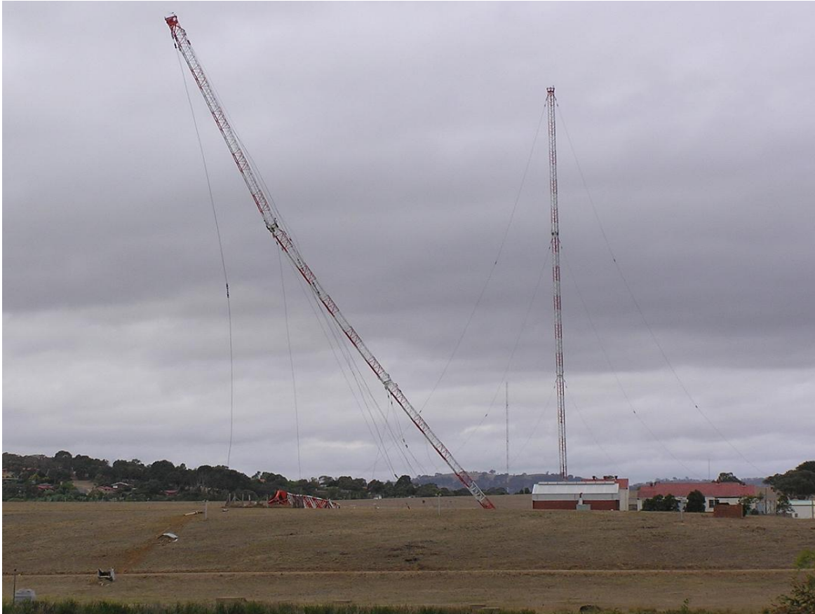
Figure 3.28 Western aerial tower at Belconnen Naval Transmitting Station being felled on 22 December 2006. (Source: Peter Ellis from Wikipedia)
