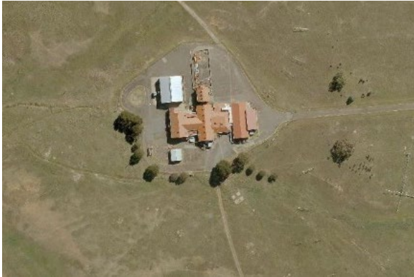
Figure 4.21 The transmitting station buildings. The large white roof is the 1972 generator building while the smaller white roof is an associated electricity substation. (Source: ACTMapi 2018)
