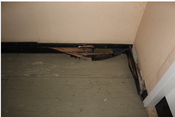
Figure 4.29 Water damaged skirting in room 13 (2018).
