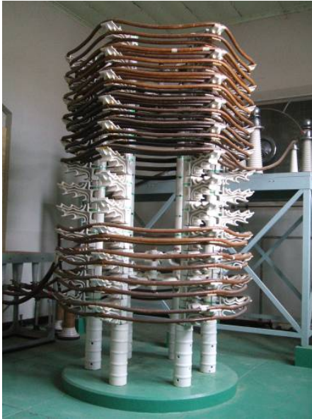
Figure 4.39 The aerial loading coil in the helix room, 2018.
