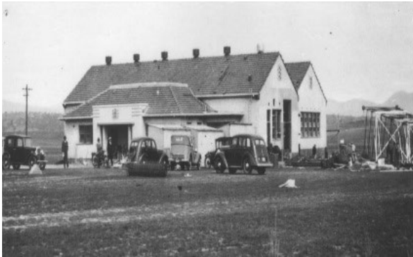
Figure 3.9 First stage of the transmitter building in early-1939. The original entry porch is visible, and the helix room is yet to be built. (Source: 2001 HA)
