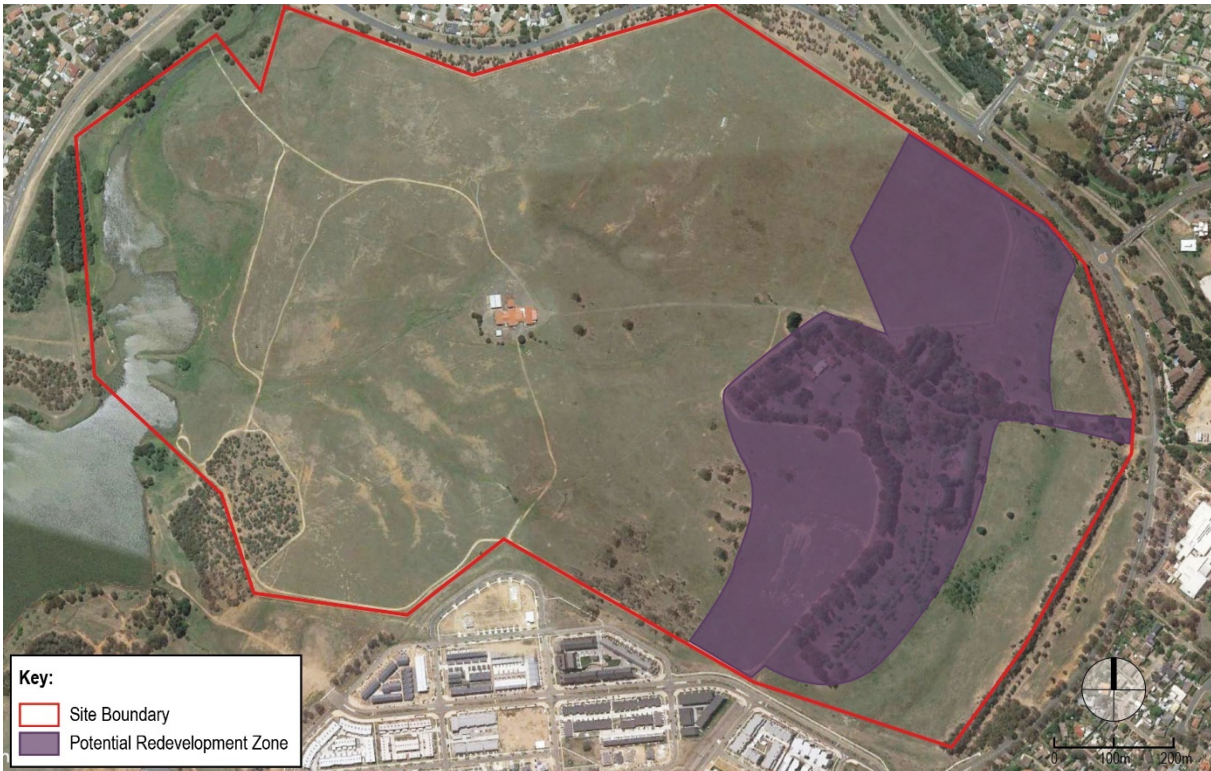
Figure 6.6 Aerial image of the BNTS site identifying a potential redevelopment zone. (Source: Google Earth with GML overlay, 2018)
