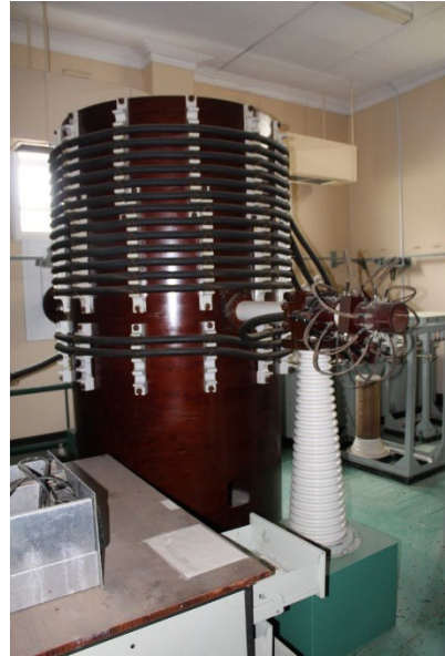
Figure 4.40 Equipment in the low-frequency transmitter room, 2018.
