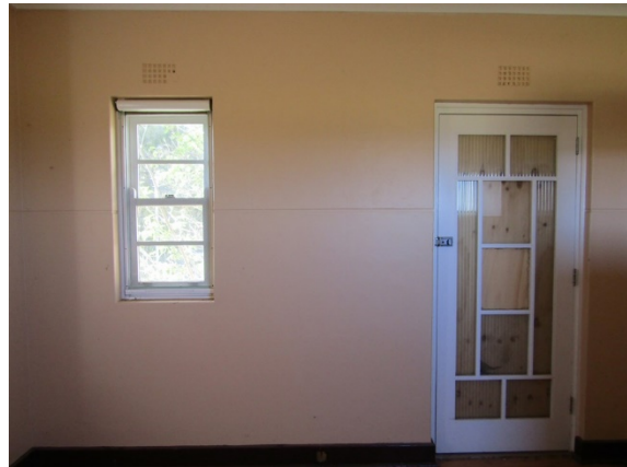
Figure 4.46 Eastern wall of second room in Guardhouse, 2019.
