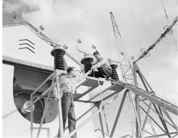
Figure 3.26 Maintenance on the aerials outside the helix room, 1961. (Source: National Archives of Australia A1200/L40032.)
