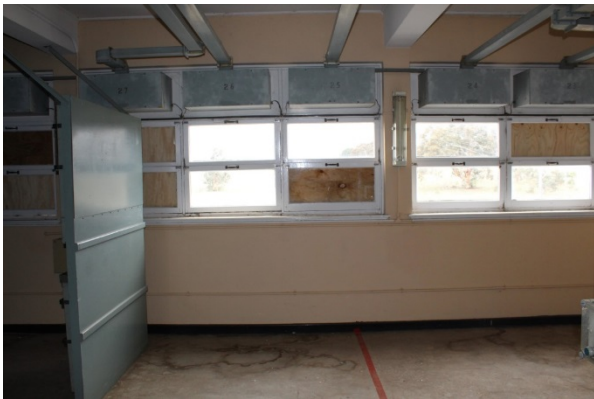
Figure 4.27 First floor Aerial Switching Room with water damage to the floor (2018).
