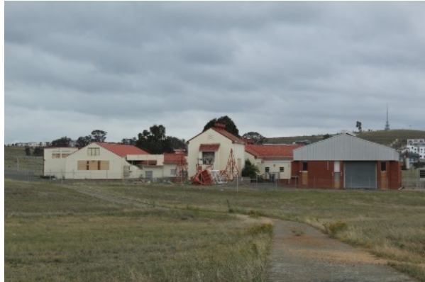
Figure 4.22 The transmitter building complex viewed looking south.
