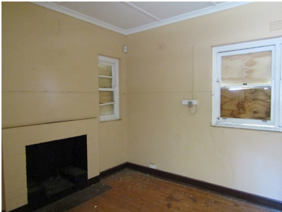
Figure 4.45 Main room within the Guardhouse. Note the boarded windows and broken glass, 2019.
