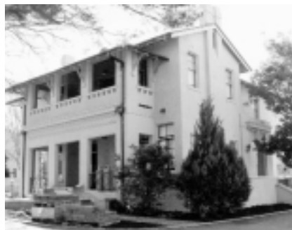
Gwynn House building after restoration in 2000.
