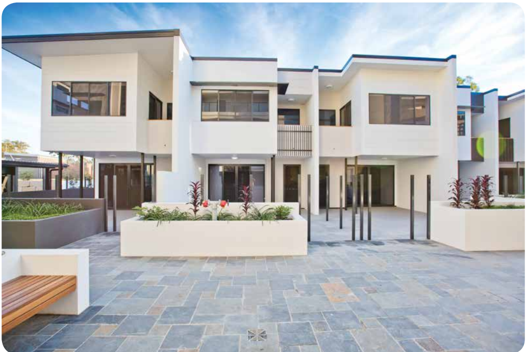
Our newly constructed apartment complex, The Landing, in Brisbane, QLD.
